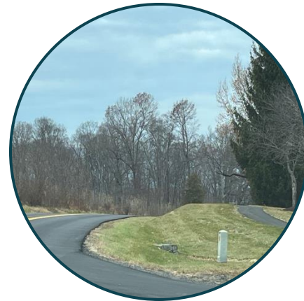
Paved (separated from traffic)
