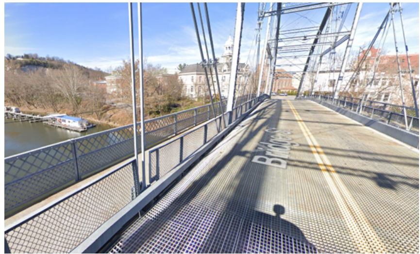
Figure 40 The Singing Bridge in Frankfort Kentucky is a historic truss bridge structure with an added cantilever bridge trail along the side for safe pedestrian and bicycle access. (Source: Google Street View)
