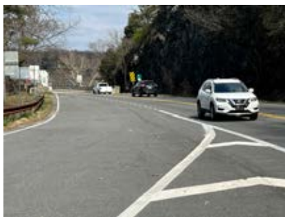
Figure 26 US 340 bridge approach at Potoma Wayside
