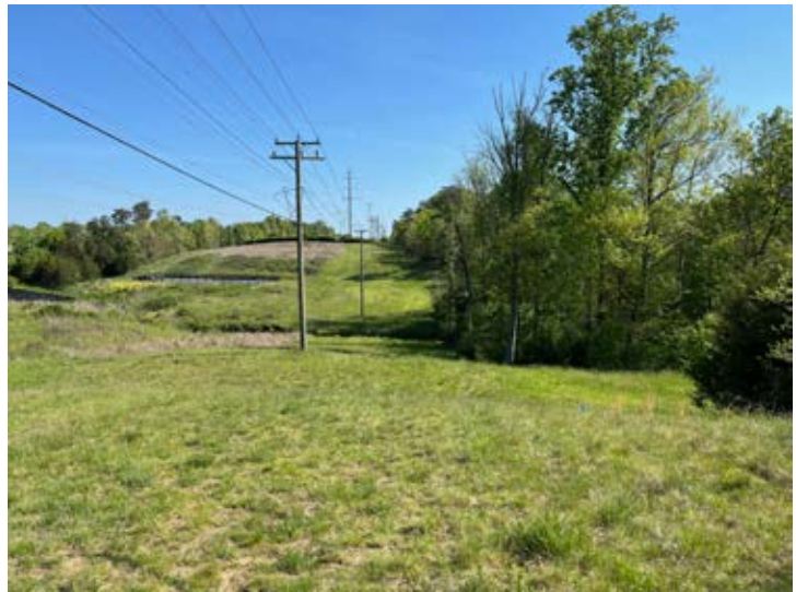
Figure 22 Constructing a trail along the edge of the overhead electric transmission line corridor would include premium costs for steep slopes and the watercourse crossing.
