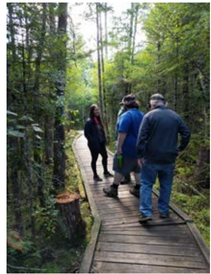
Figure 49 Example of single track boardwalk built to preserve sensitive natural features at Silver Lake Preserve, NY (The Nature Conservancy)
