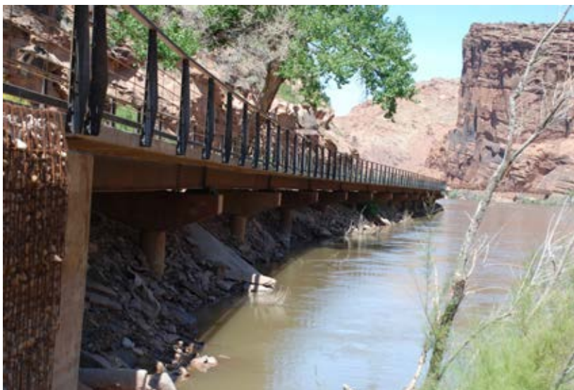
Figure 44 Example of cantilevered trail on shoreline of Colorado Riverway Trail near Moab, UT
