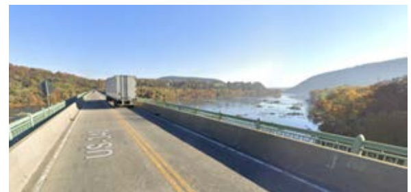
Figure 29 US 340 bridge over the Potomac River existing conditions (Source: Google Street View)
