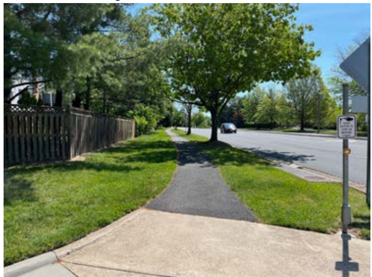
Figure 23 Widening the existing asphalt path along Balls Bluff Road may incur premium costs if the curb and gutter system need to be modified.
