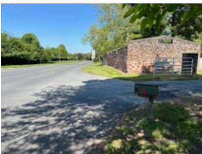
Figure 4 Example of segment with limited feasibility along Edwards Ferry Road at Red Rock Overlook Regional Park
