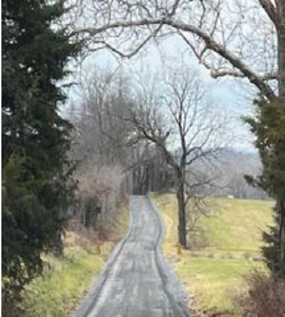
Figure 30 Featherbed Lane is an example of a low volume, unpaved road considered for designation
