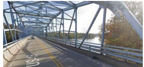
Figure 28 Point of Rocks Bridge (Source: Google Street View)
