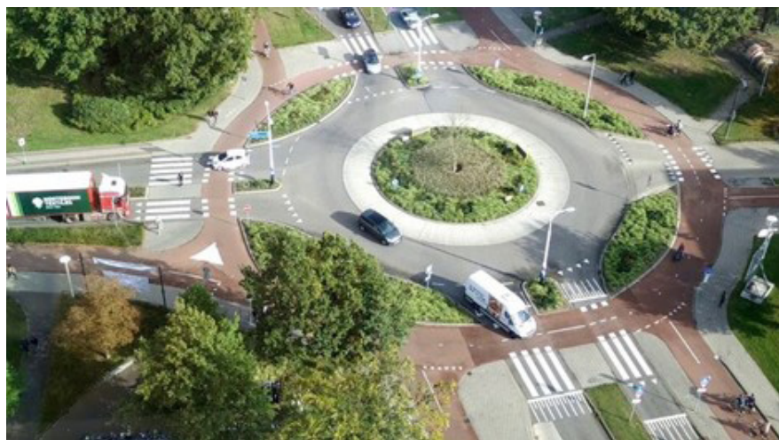
Figure 46 Example roundabout with separated, dedicated space for pedestrian, bicycles, and vehicles (Source: Car Free America)
