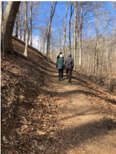
Figure 48 Example of bench cut trail in Fountainhead Park (NOVA Parks)
