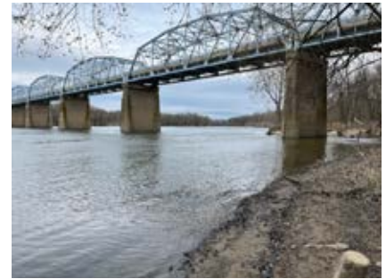
Figure 33 McKimney Boat Ramp at Point of Rocks bridge
