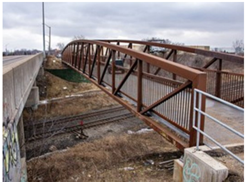
Figure 41 A parallel and separate prefabricated pedestrian bridge adjacent to a roadway bridge.
