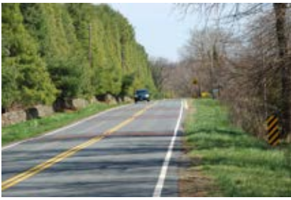
Figure 35 Textured pavement warning strips with spacing that decreases approaching Upperville with introduction of flush curb to signal to drivers to slow down
